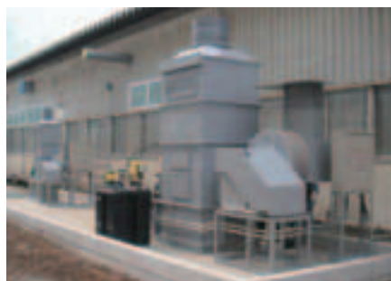
Moisture-type exhaust gas scrubber (installation example)
